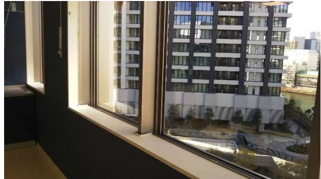
Figure 6.Example of construction of antiviral PVC sheet by Sy (window frame of hospital)
